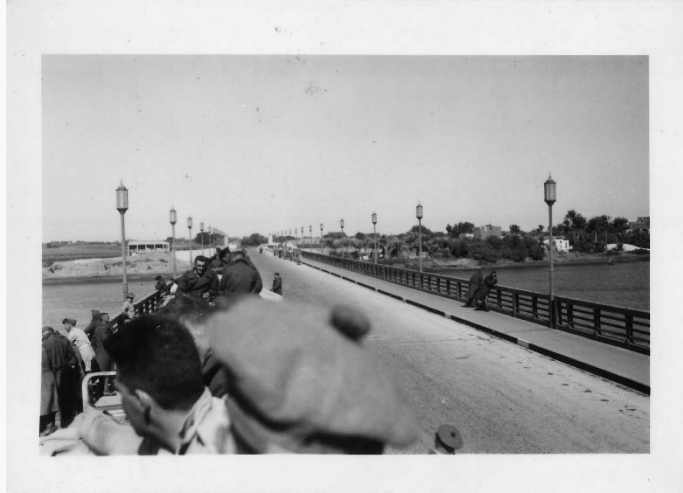
4 th October 1941 Bridge over Nile at Tanta
