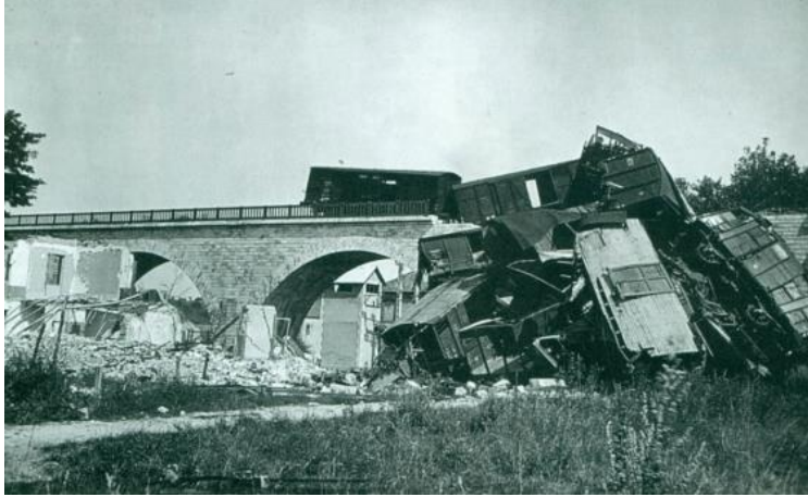
The Gien railroad bridge, after 1940 battle
